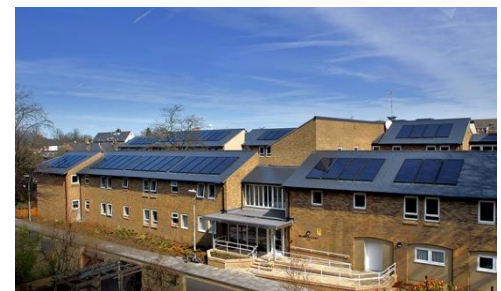
Roof integrated solar photovoltaics, Brandon Court, Cambridge
