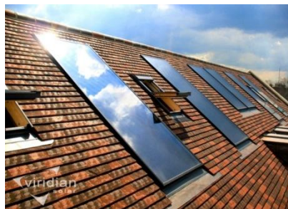
Installation of solar thermal panels Paradise Street, Cambridge
